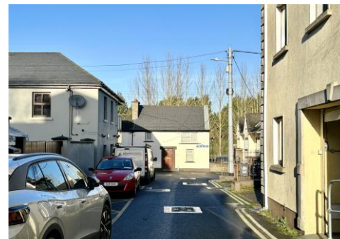
Figure 4.14 Lack of Footpath on Kelly’s Lane
