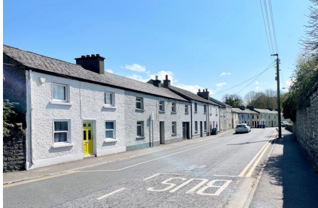
Figure 8.1 Vernacular Built Heritage on Parson’s Street
